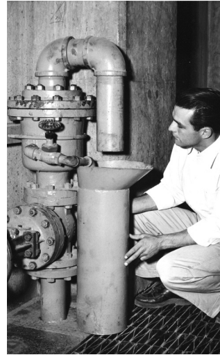
Circa 1940, a Crispin Air Valve installed on the Hoover Dam
